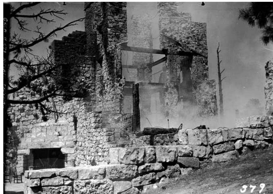
The original Grand Canyon Lodge's outside fireplace and stairwell smolder in ruins after being destroyed by a kitchen fire in 1932.
